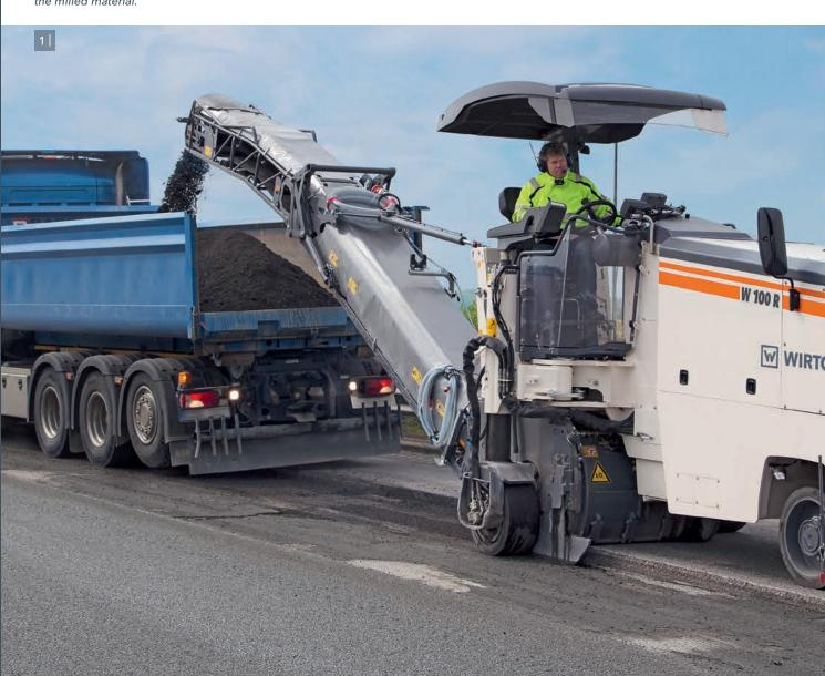
1 | The small milling machine features high-performance, efficient loading of the milled material.
